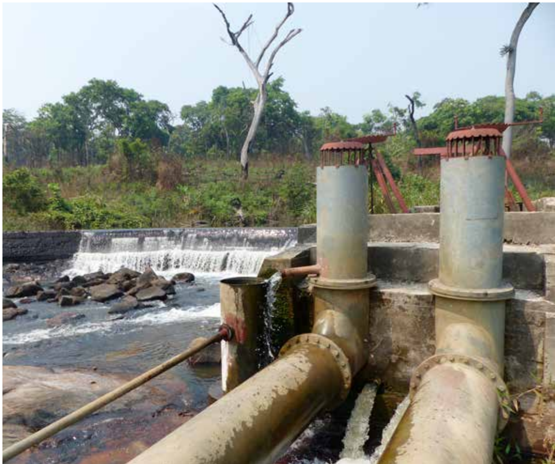
The dam built for the ELKAP project, where the penstocks provide water to the turbine station.
