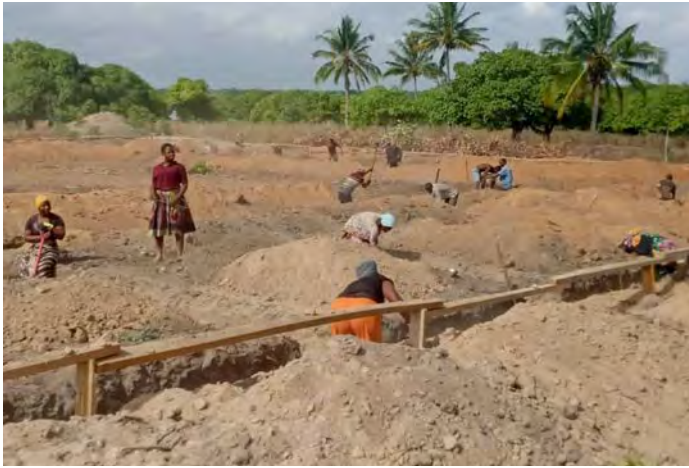
Trenches are being dug to lay the foundation
