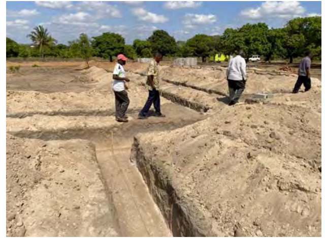
Trenches are being dug to lay the foundation
